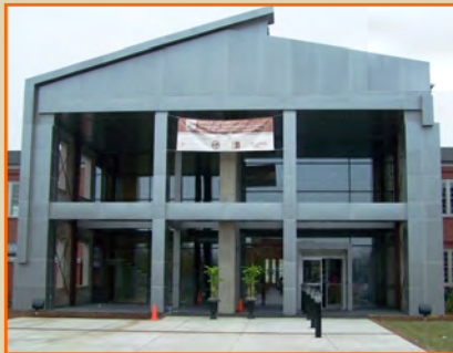
Above - Main entrance to the James E. Clyburn Intermodal Transportation Center in Sumter, before (top photo) and after (bottom) renovation. Photos by Ann August
